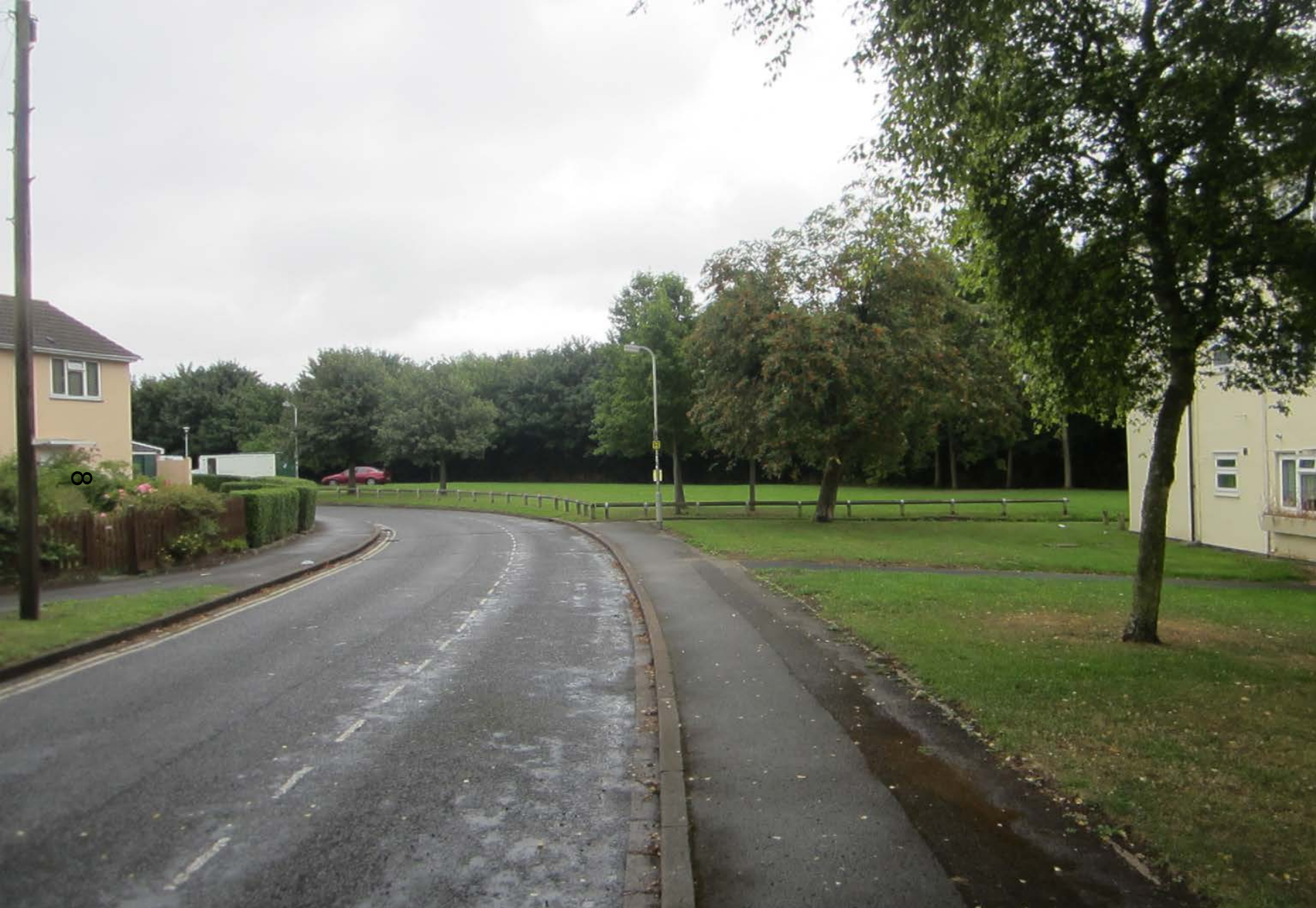
View of site looking northwards along Warren Crescent
